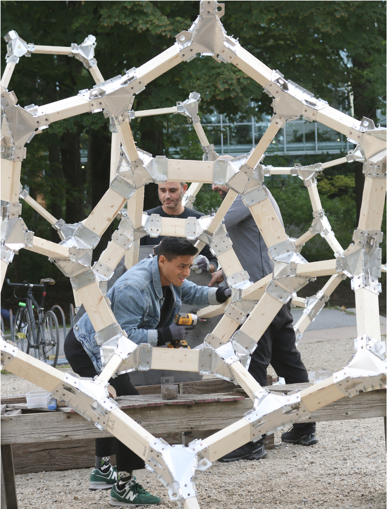
5 Applying the finishing touches on one of the structural legs (Kevin Larouche-Wilson, © 2022).
